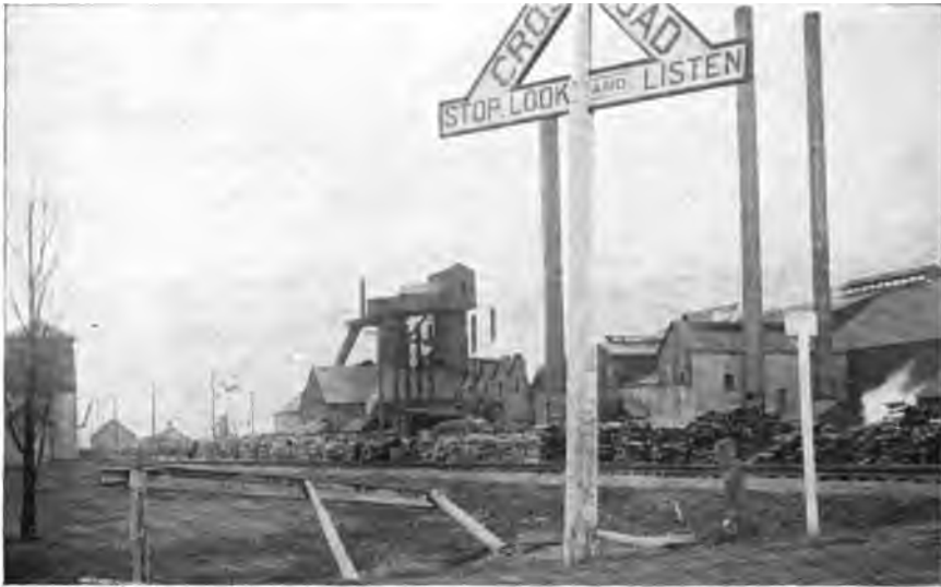
A. ANTRIM IRON FURNACE.
